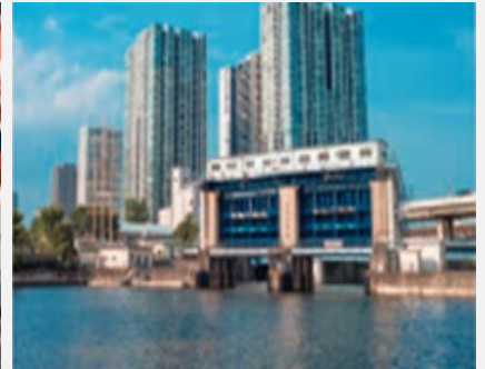
Flood gate monitoring
